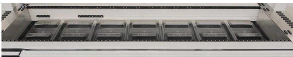
Fig. 20: Deck trays beneath the deck segments
