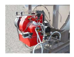
The control panel includes indicators inlet and outlet water temperature, temperature of flue gases, switches for boot pumps and burner. The Equipment has protection systems for both lack of pressure in the circulation system as excess pressure, and an extra temperature control emergency programmed to cut off power of the burner in case of failure of the control (pyrometer) starting and stopping.
