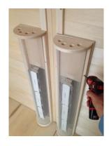
Flush mounted heaters on the back wall have the flush-mounted screens.
