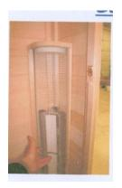
The Heat protection Screens are mounted with the holes Upward to the top. Screw the screen onto the wall with only one inch clearance on the bottom, and maximum clearance on top, to allow heat dispersion.
