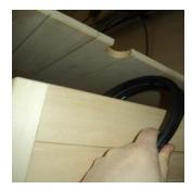
The Front ceiling piece has a "notch" to allow the cables from the control panel to slide up and onto the roof for connection. All other cables should be flung up and over the walls in the corner to allow the roof to fit on.
