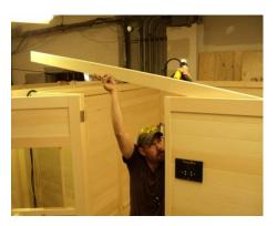
The "Header" board is screwed on from the inside. The holes are pre-drilled.
