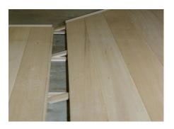
The Two pieces are designed with slats that inter-lock. A grooved rail is on either side.
