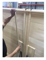
The long thin pieces screw onto the Back and Front of the back wall to hold the two side panels together. They are marked UP and DOWN on the under side.
