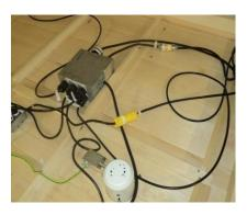
All cords connect to Grey Box on rooftop. 6 Heaters plug into oneside. Controller cables are different and plug in next to each other on the opposite side.
